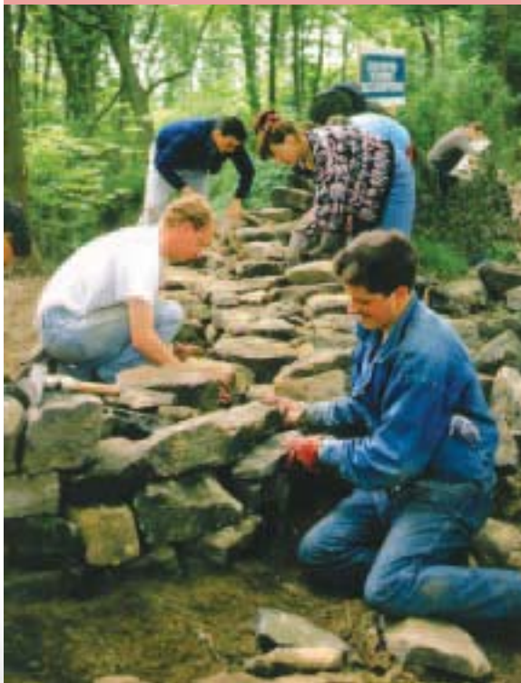
Figure 12 Volunteers working on a dry stone wall at Outwoods.
